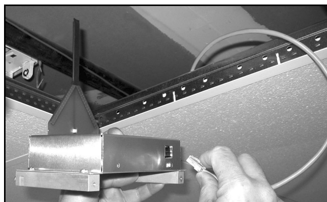
FIG. 1: AFTER SECURING ANTENNA, PLUG THE ETHERNET CABLE INTO THE REAR RJ-45 SOCKET.
